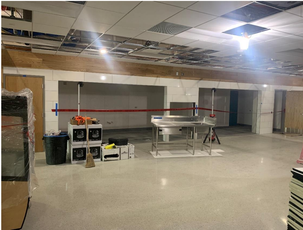
19. Area 5 – Epoxy flooring install in servery in progress.
