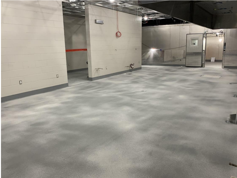
10. Area 3 - Epoxy flooring install in the culinary lab in progress.
