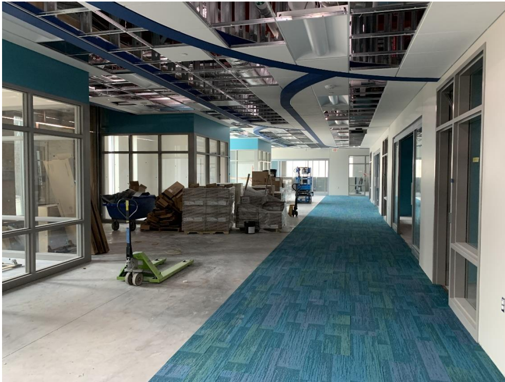
12. Area 4 – Corner guard and window sill install in progress throughout gradewing area.
