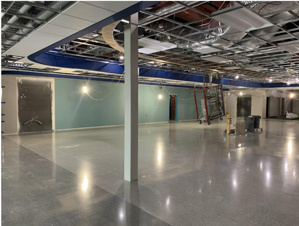
16. Area 3 – Terrazzo flooring in corridor appears to be installed. Dimensional letters at feature wall appear to be installed.
